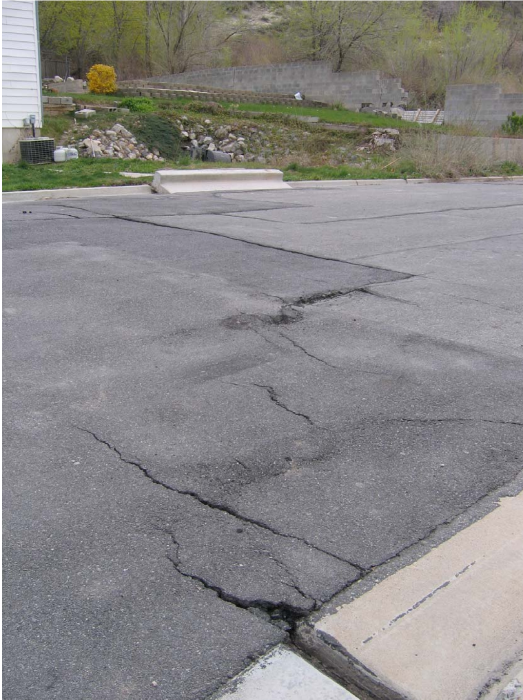
Figure 4. Road damage to south end of Springhill Drive along south-flank shear zone. View is upslope and to the southeast. Tilted and displaced curb and gutter visible on opposite side of road. Ground on left side of photograph is moving downslope (toward bottom-left edge of photograph). Photograph taken in May 2008.
