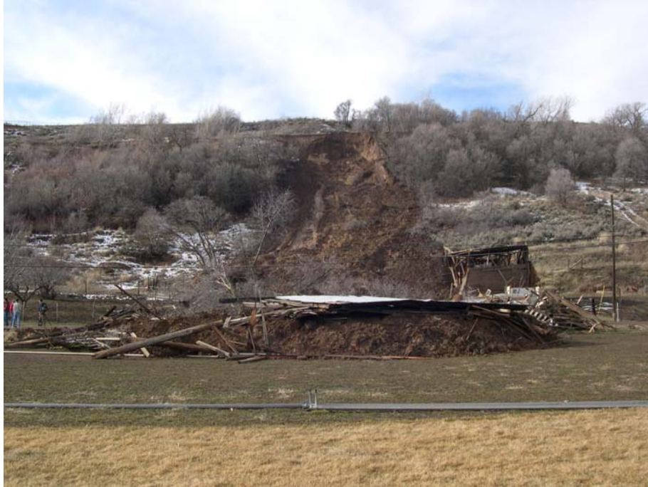
Figure 2. View to the south showing the landslide main scarp in the Davis-Weber Canal embankment, the demolished barn (right foreground), and runout onto the field.
