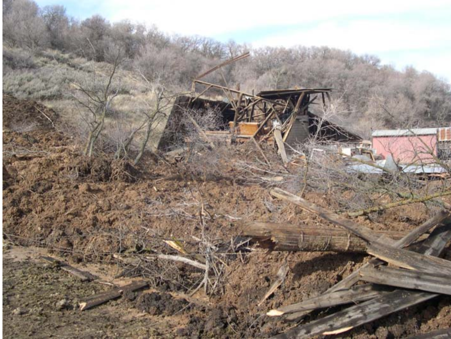
Figure 4. Looking across the lower part of the landslide at the demolished barn. The clump of trees in the foreground was rafted downslope on top of the landslide debris.
