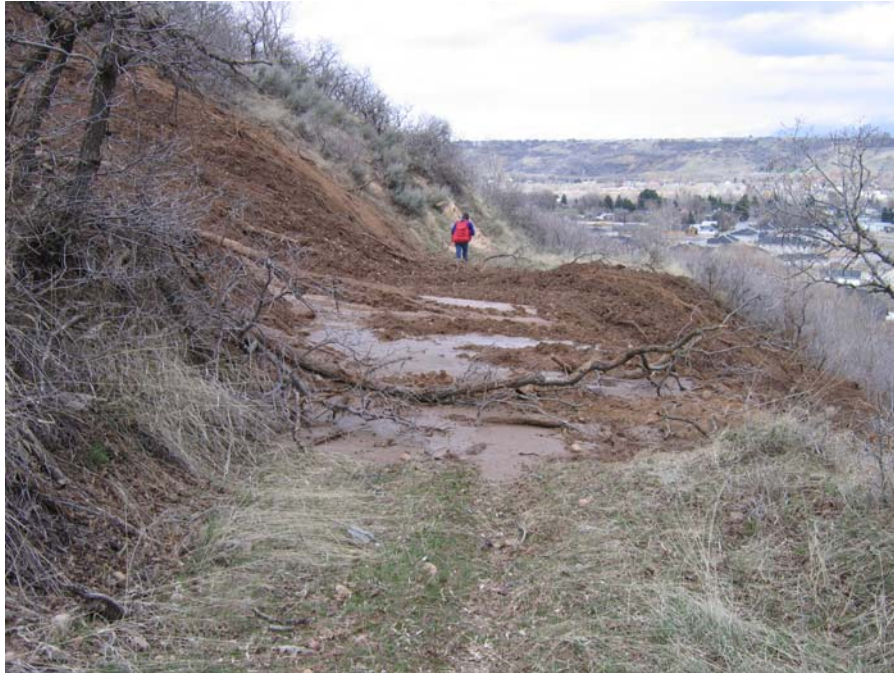
Figure 10. Landslide material deposited on a dirt road midslope above the Davis-Weber Canal.
