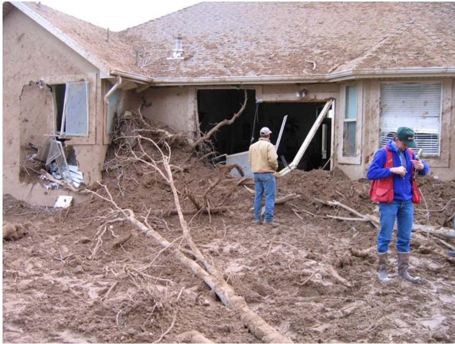
Figure 3. Landslide damage to the house at 1650 East 7687 South.
