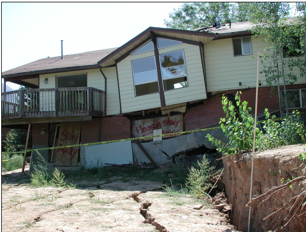
Figure 2. Damage to one of three houses destroyed by movement of the Heather Drive landslide, Layton in 2001.
