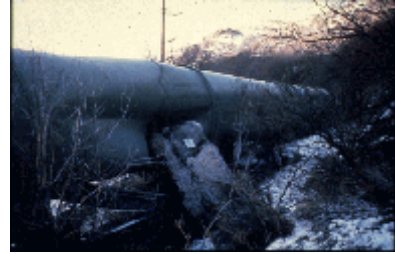
Olmstead Aqueduct damaged by rock fall. Photograph by Robert Robison, Utah County Geologist.
