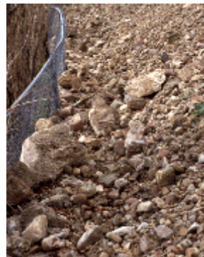
Rocks accumulated behind a chain-link fence.
