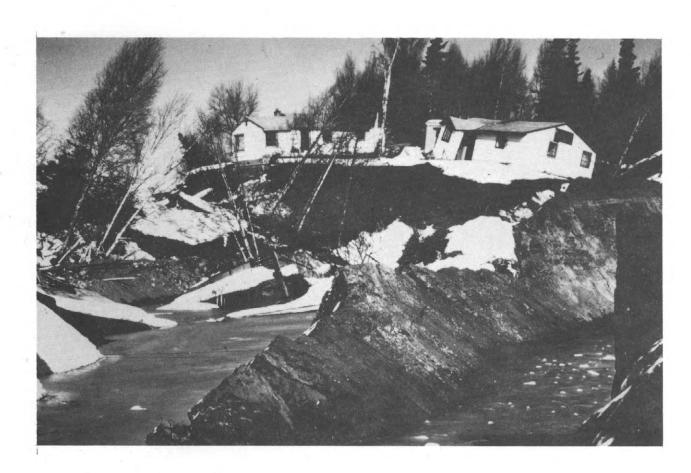
FIGURE A-4 Earthquake damage resulting from ground failure. Turnagain Heights landslide, Anchorage, Alaska, March 27, 1964.
