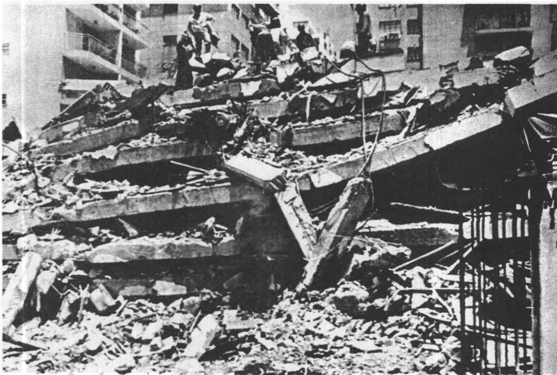
FIGURE A-4. Mijagual high-rise apartment building in Caracas, Venezuela, showing total pancake collapse.
