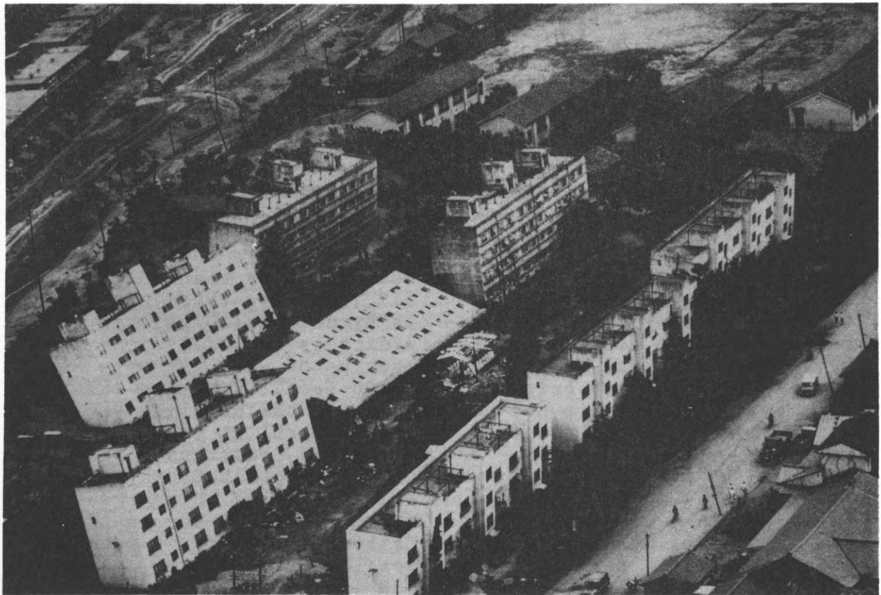
FIGURE A-6. Earthquake damage resulting from ground failure: Liquefaction. Niigata, Japan, 1964.
