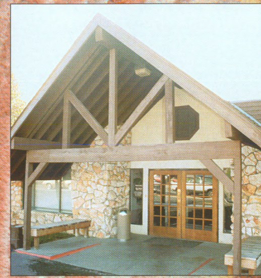
Vejo rhyolite (rainbow variety) rubblestone veneer, on the St. George Care Center, St. George, Utah.
