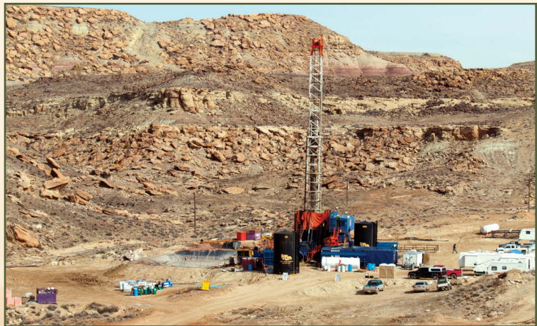
Drilling operations, Greater Aneth field, San Juan County
