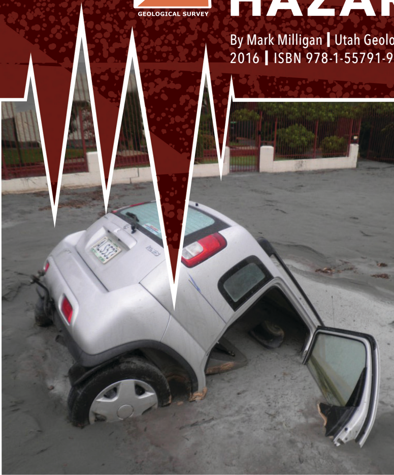
A small car presumably sunk into a large sand blow on a road damaged by liquefaction during the 2011 Christchurch, New Zealand, earthquake. In this extreme example, sand covered the road due to ground-surface subsidence and sand blows. Image courtesy of Mark Lincoln.
