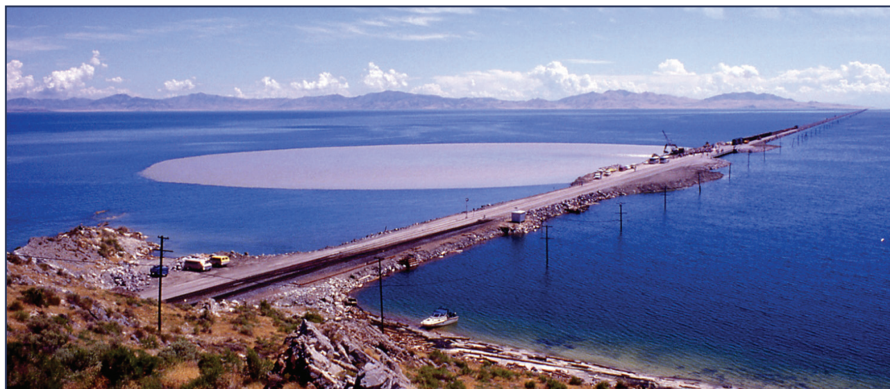
The 290-foot breach of 1984 at Lakeside. The 3.5-foot head differential in lake elevation between the north and south arms caused a surge of water to the north, stirring up sediment from the lake floor (light-colored circle in lake). View is to the northeast. The Promontory Mountains are on the horizon. UGS file photo.
