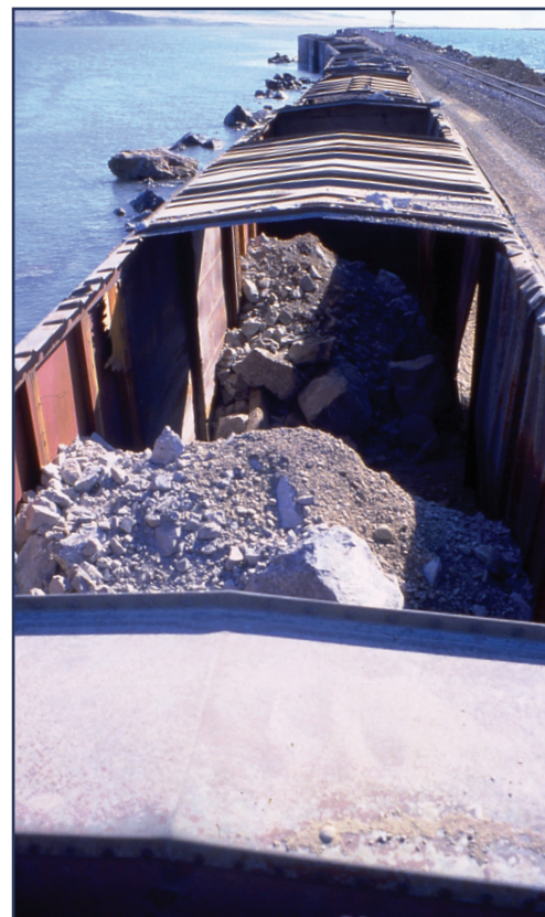
Construction of the Boxcar Seawall, September 1983. The middle one-third of the tops of the cars were removed so they could be loaded with rock. UGS file photo.
