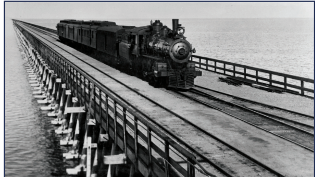
The 12-mile Lucin Southern Pacific trestle, circa 1906. The trestle necessitated more than 38,000 piles (clusters of five trestle pilings per 15 feet) of Douglas fir, ranging from 80 to 130 feet long, driven into the soft mud of the lake bottom, decked with redwood, and topped with gravel. Photo courtesy of the Utah State Historical Society.
