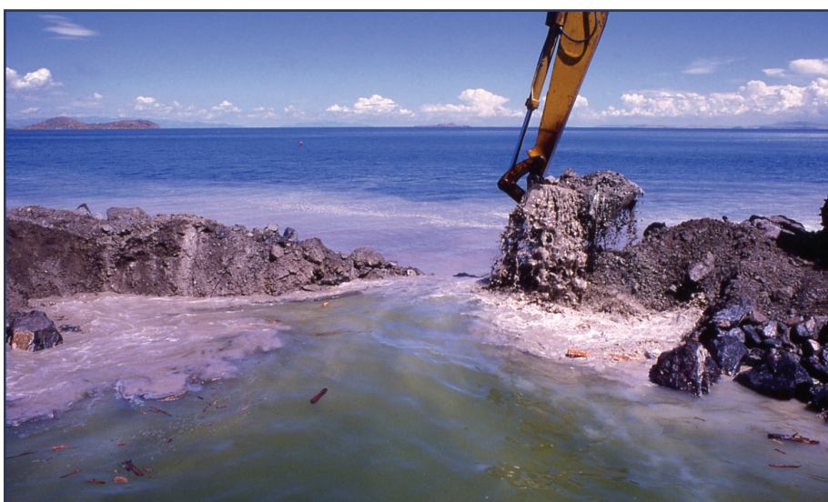
The last scoop breaching the causeway in August 1984 at Lakeside to alleviate flooding in the south arm. View is to the north, Gunnison Island at upper left horizon. UGS file photo.
