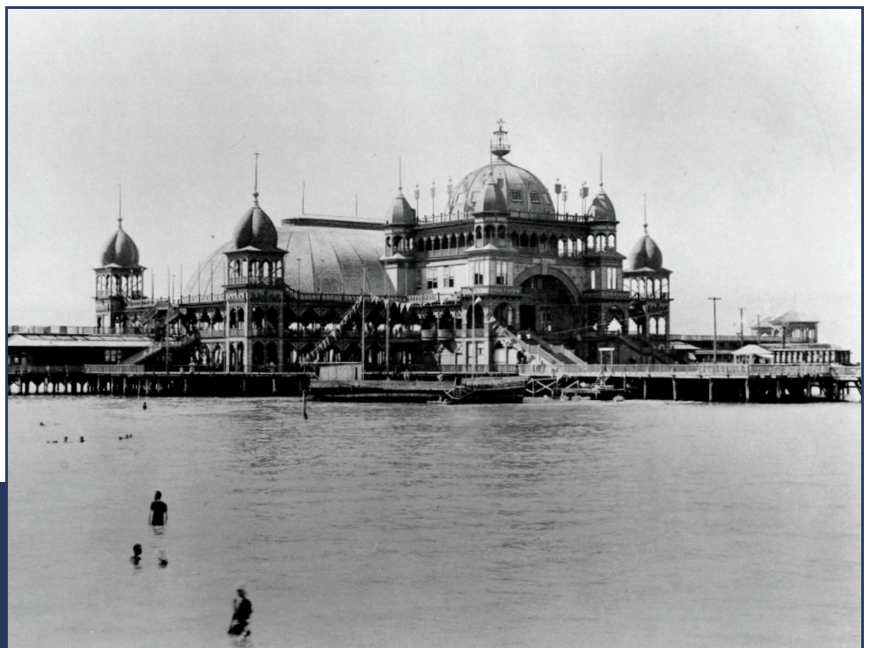
Saltair in 1896. Two thousand pilings were used to elevate the structure above the fluctuating lake level. Throughout the three Saltairs’ history the lake has flooded and retreated from the resort. Photo courtesy of the Utah Division of State History.
