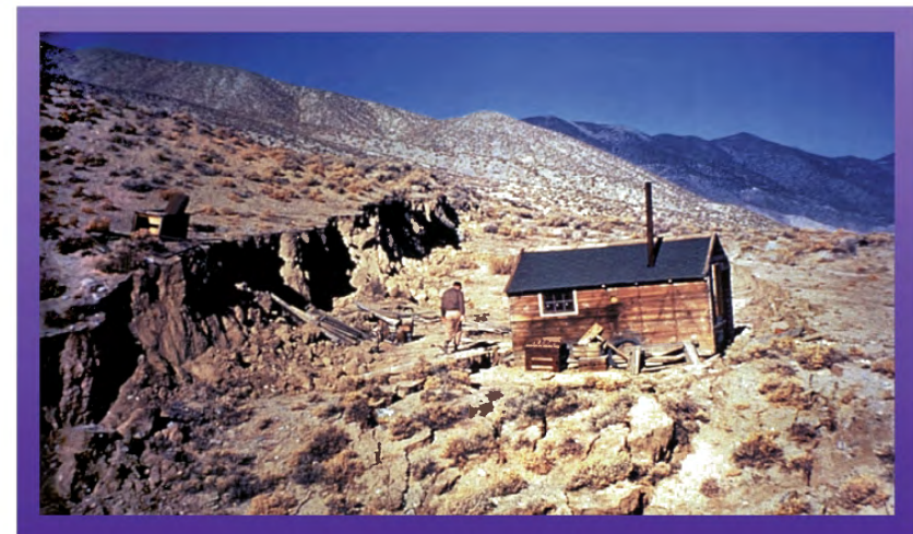
Tilting and cracking of the ground surface on the down-dropped side of a fault (1954, magnitude 6.8 Dixie Valley, Nevada earthquake).
