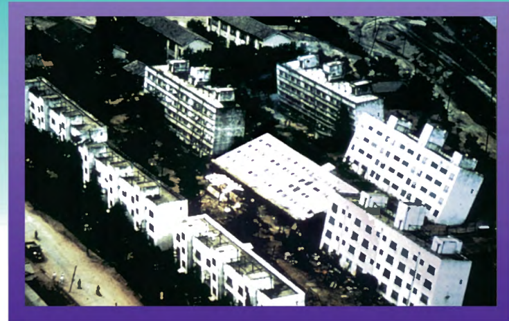
Liquefaction caused these apartment buildings to tip over during the 1964, magnitude 7.4 Niigata, Japan earthquake (Earthquake Engineering Research Institute).
