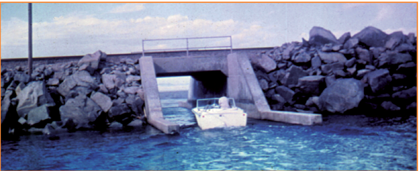
One of the two 15-foot-wide by 20-foot-deep culverts in the rock-fill portion of the causeway. Photo taken during low lake level (1960-1962).
