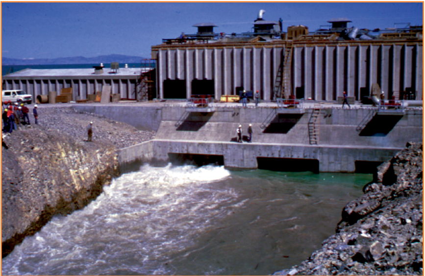
Close-up view of the pumping plant with one of the three 1,000 cubic-feet-per-second pumps in operation (view looking east).
