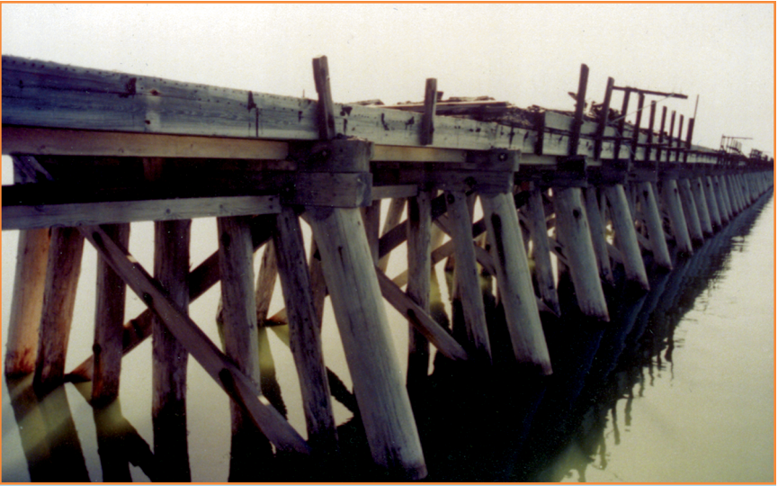
Original wooden trestle railroad that crossed Great Salt Lake, constructed about 1903. Photo by June Cannon, Cannon Structures, Inc.. A salvage operation for the wood started in 1993; some is used in the lobby of the Department of Natural Resources building.
