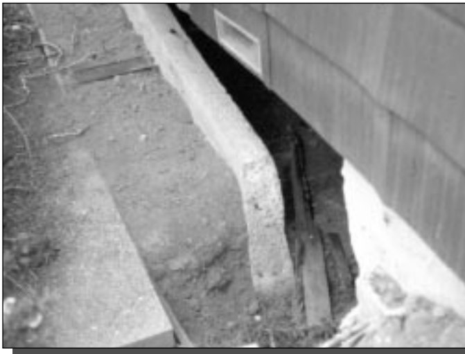
Foundation Damage
