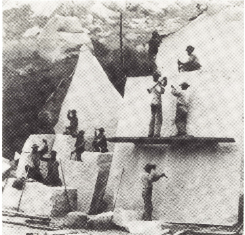
Quarried stone was used to build many of Utah's historic structures. This photo of the Little Cottonwood Canyon quartz monzonite quarry shows workers cutting large blocks from massive rock walls. The blocks were later wedged into more desirable sizes. Photo courtesy Utah Historical Society.
