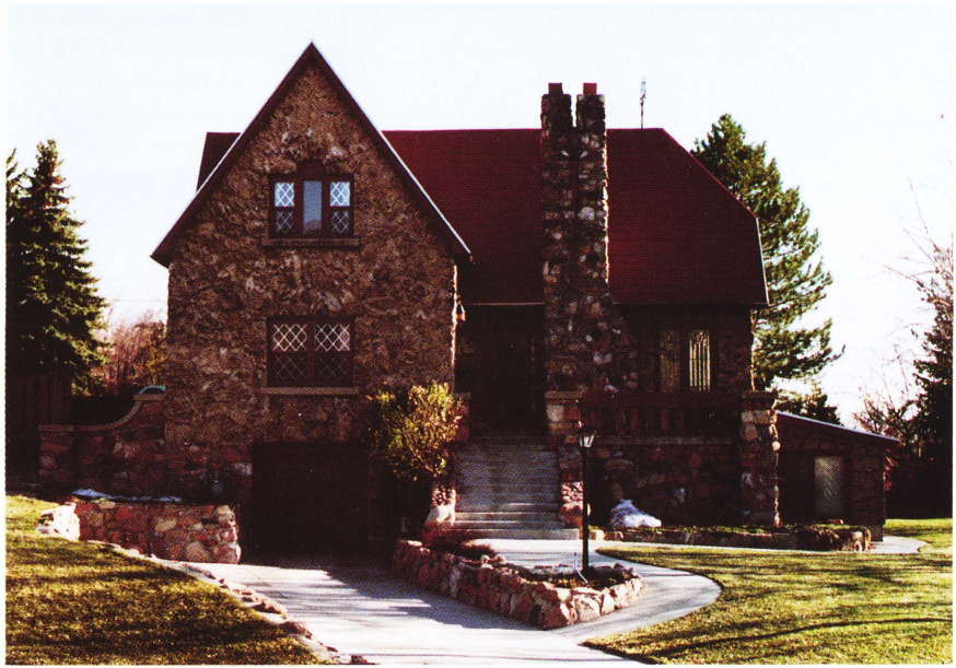
Everyone depends on natural resources. Our cars, bicycles, computers, almost everything we use is made with the earth's assets. This home was constructed with volcanic rocks from Wasatch County and Nugget Sandstone from Salt Lake County. Clay was used for mortar and in the sidewalks.
