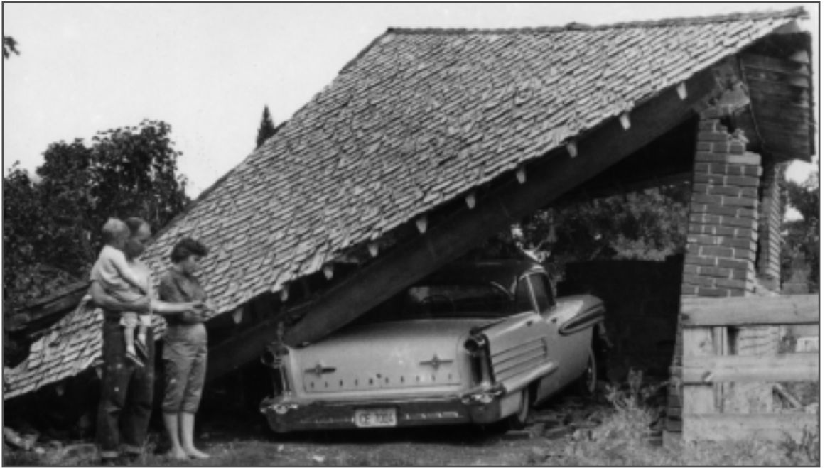
This brick garage collapsed onto a car in Richmond.
