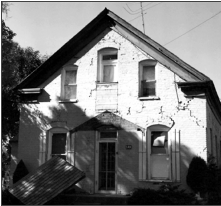
Cracked walls and fallen porch contributed to the decision to tear down this home.
