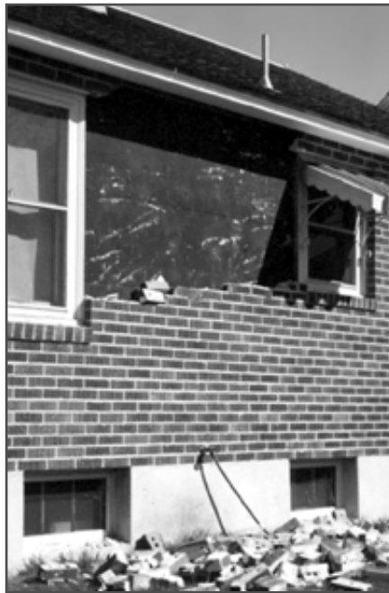
The brick veneer fell off part of this house.
