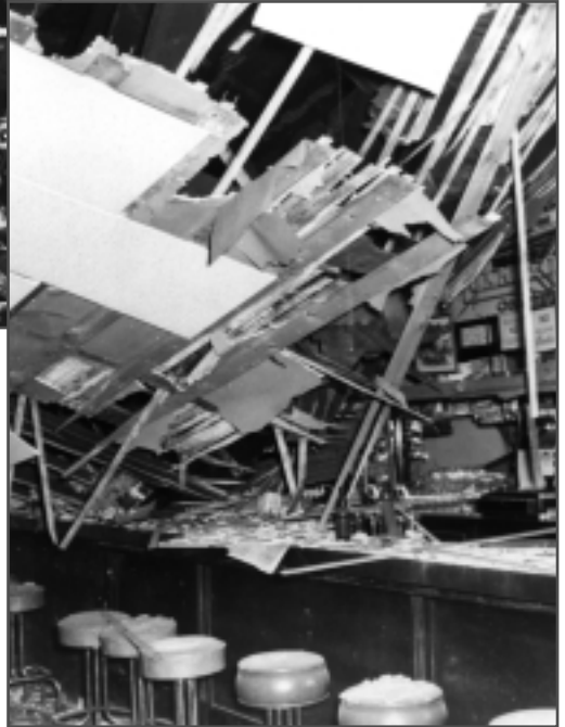
Right: The walls spread apart inside the Model Billiards building in Logan, allowing the roof to fall.
