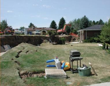
The cause of the 2001 Heather Drive landslide movement is unclear. Other nearby landslides reactivated in 1998 as the result of above-normal precipitation and elevated ground-water levels.
