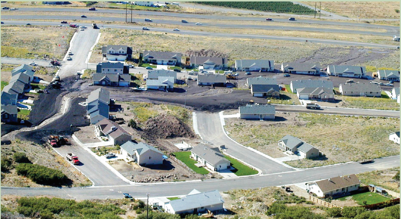
The 2002 Santaquin debris flow traveled through this subdivision, damaging houses, burying streets and lots, and depositing sediment (view to the west). Photo by Dale Deiter, U.S. Forest Service.
