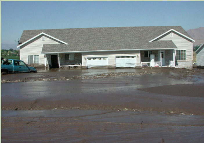
The 2002 Santaquin debris flow broke through the door at the left, deposited sediment in the house, buckled garage doors, partially buried vehicles, and buried streets and lots.
