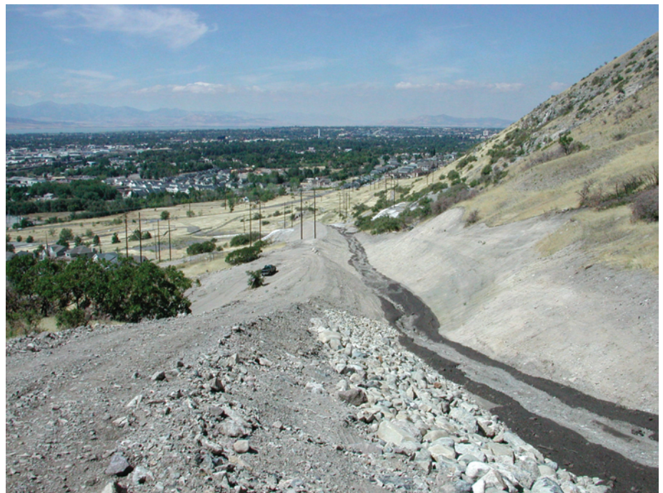
Example of a protective structure that turned the debris flow (in the channel) away from houses (at left) in Provo.
