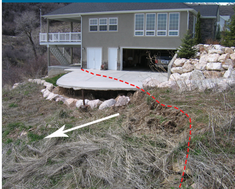
The red line defines the upper edge of a Creekside Drive area landslide (located on Cascade Drive) that partly underlies a driveway slab. White arrow indicates direction of movement. Landslide movement left the slab unsupported.
