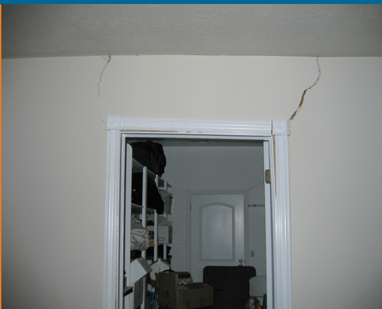
Landslide movement caused severe structural damage to this house (located on Creekside Drive), including cracks in the walls and foundation. The nature and extent of damage led the owner to abandon the house in April 2006.
