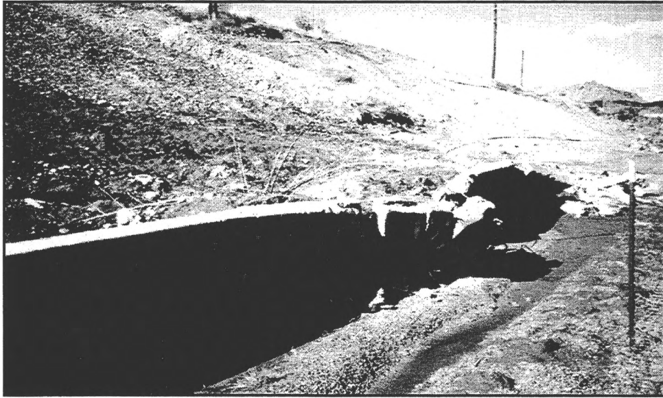
Attachment 7. Broken retaining wall at the toe of the Santa Clara Little League field landslide (north end); water draining from the landslide is flowing in a shallow ditch in front of the wall.
