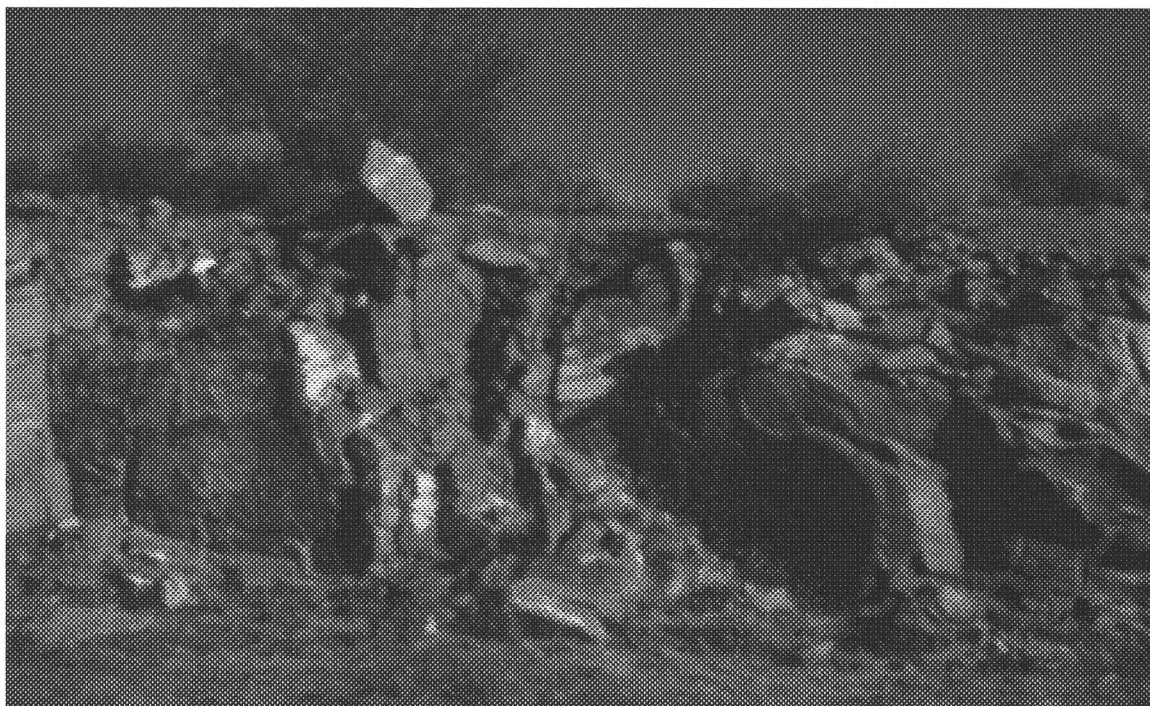
Attachment 6. Close-up of jointed Navajo Sandstone exposed in construction cut on Winchester Hills Phase 8. View is to the southeast.
