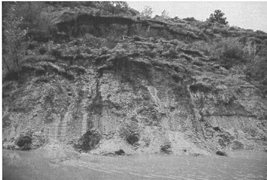
Attachment 3. South views of shallow earth sliding on the right (eastern) flank of the 1998 landslide in South Weber on May 1 (top) and May 11 (bottom). The Davis-Weber canal is in the foreground.
