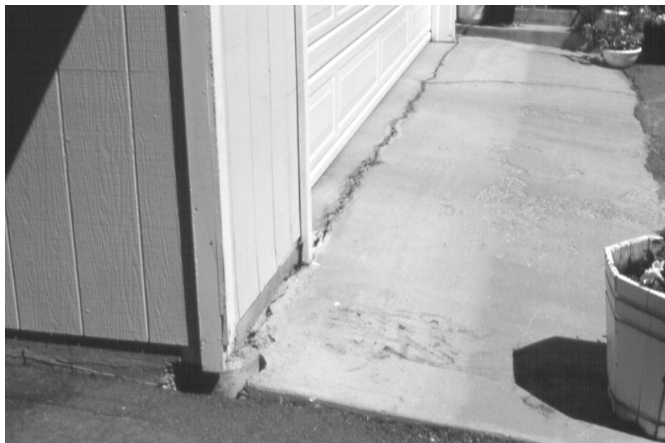
Attachment 3. Porch (top) and driveway (bottom) at 592 South showing cracks and eastward tilting of concrete.
