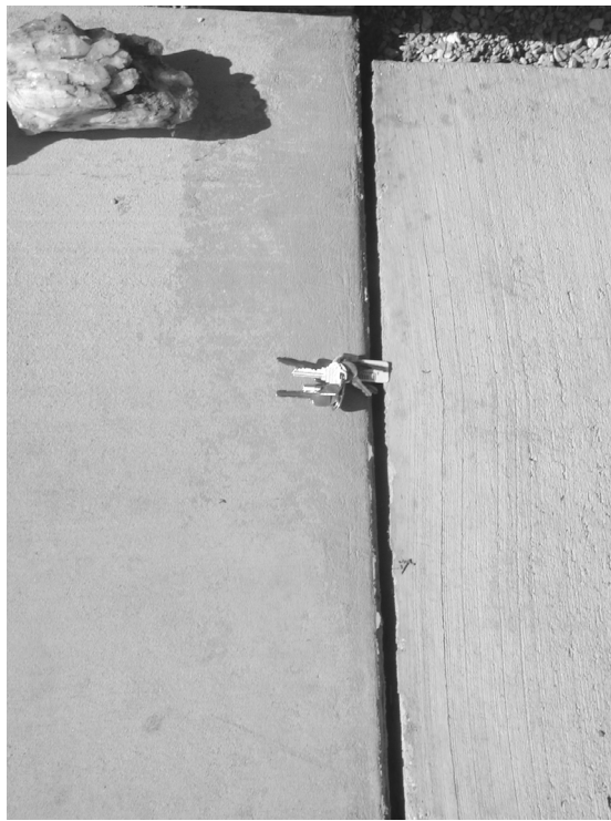
Figure 2. Pull apart between sidewalk as the slab on the left moves to east.
