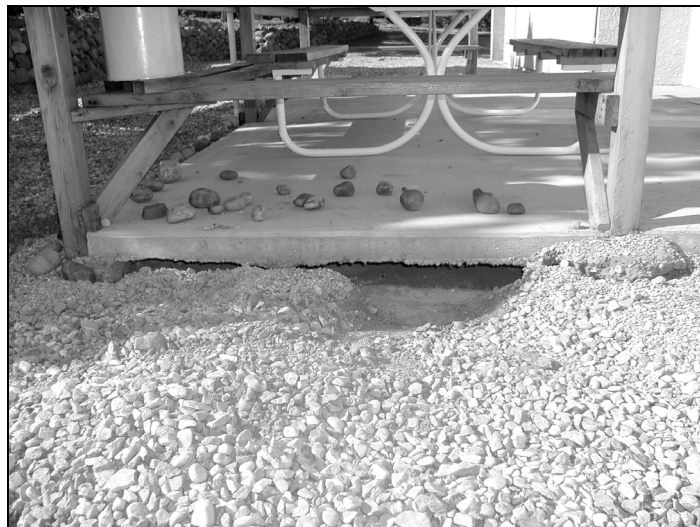
Figure 6. Void space beneath concrete patio slab due to soil collapse. View to the south.
