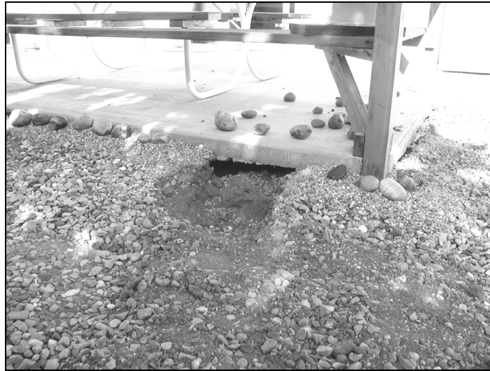
Figure 7. Void space beneath concrete patio slab due to soil collapse. View to the west.
