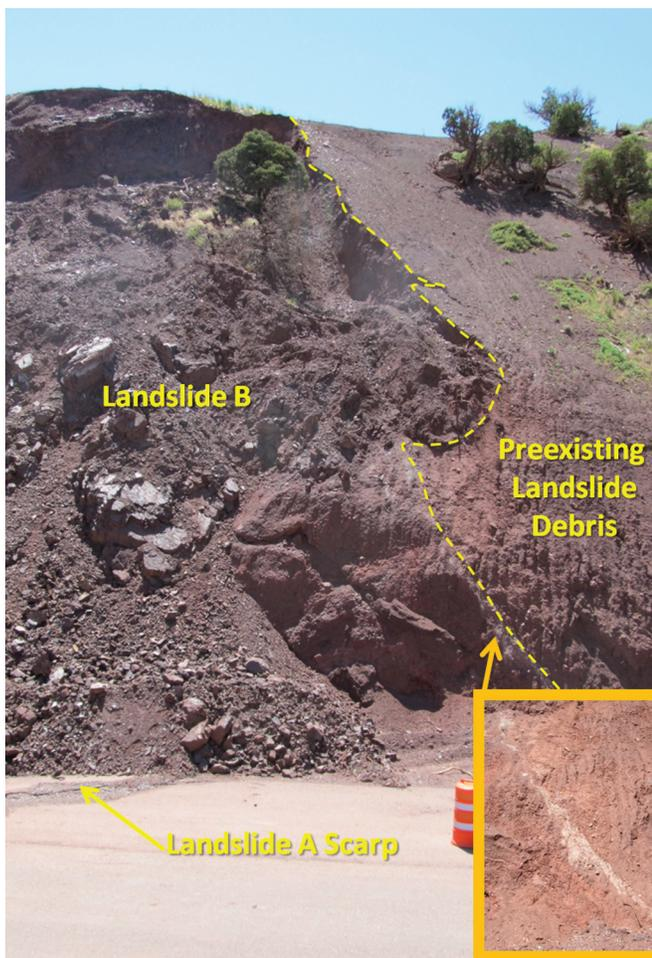
**Figure 6.** Contact between Landslide B and preexisting landslide debris. Exposure in western road cut slope along Browns Park Road. Inset shows discoloration of material along right flank shear plane of preexisting landslide low on cut slope. Photo taken on June 21, 2011.
