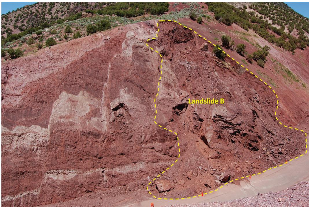
**Figure 4.** Western cut slope of roadway through cut showing Landslide B. Browns Park Road with one lane blocked in the foreground. Bedrock is Upper Jesse Ewing Canyon Formation shale and silty sandstone. Numerous steeply dipping normal faults are marked by offset of light-colored beds in left part of photo. Photo taken on June 21, 2011.
