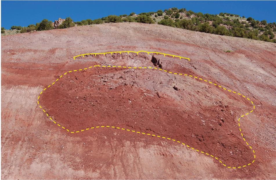
**Figure 10.** Landslide C main scarp and deposits on road cut slope. Hachured yellow line marks main scarp and dashed yellow line shows approximate boundary of landslide deposits. Photo taken on June 22, 2011.
