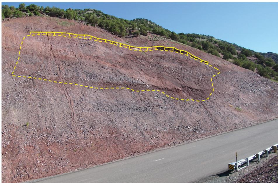
**Figure 13.** Landslide E on upper part of road cut slope. Yellow hachured line marks main scarp and dashed line shows approximate boundary of landslide deposits. Photo taken on June 22, 2011.
