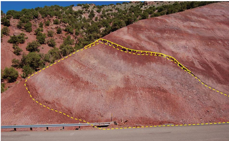
**Figure 11.** Landslide D main scarp and a part of its deposits on road cut slope. Landslide deposits filled a small roadside ditch and covered a portion of a guardrail. Hachured yellow line marks main scarp and dashed line shows approximate boundary of landslide deposits. Photo taken on June 22, 2011.
