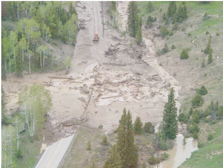
Figure 8. View northwest of SR-14 blocked by sediment from the Black Mountain debris flow. Crow Creek is on the right. Photo taken on June 3, 2005, by Lt. David Excel, Utah Highway Patrol.
