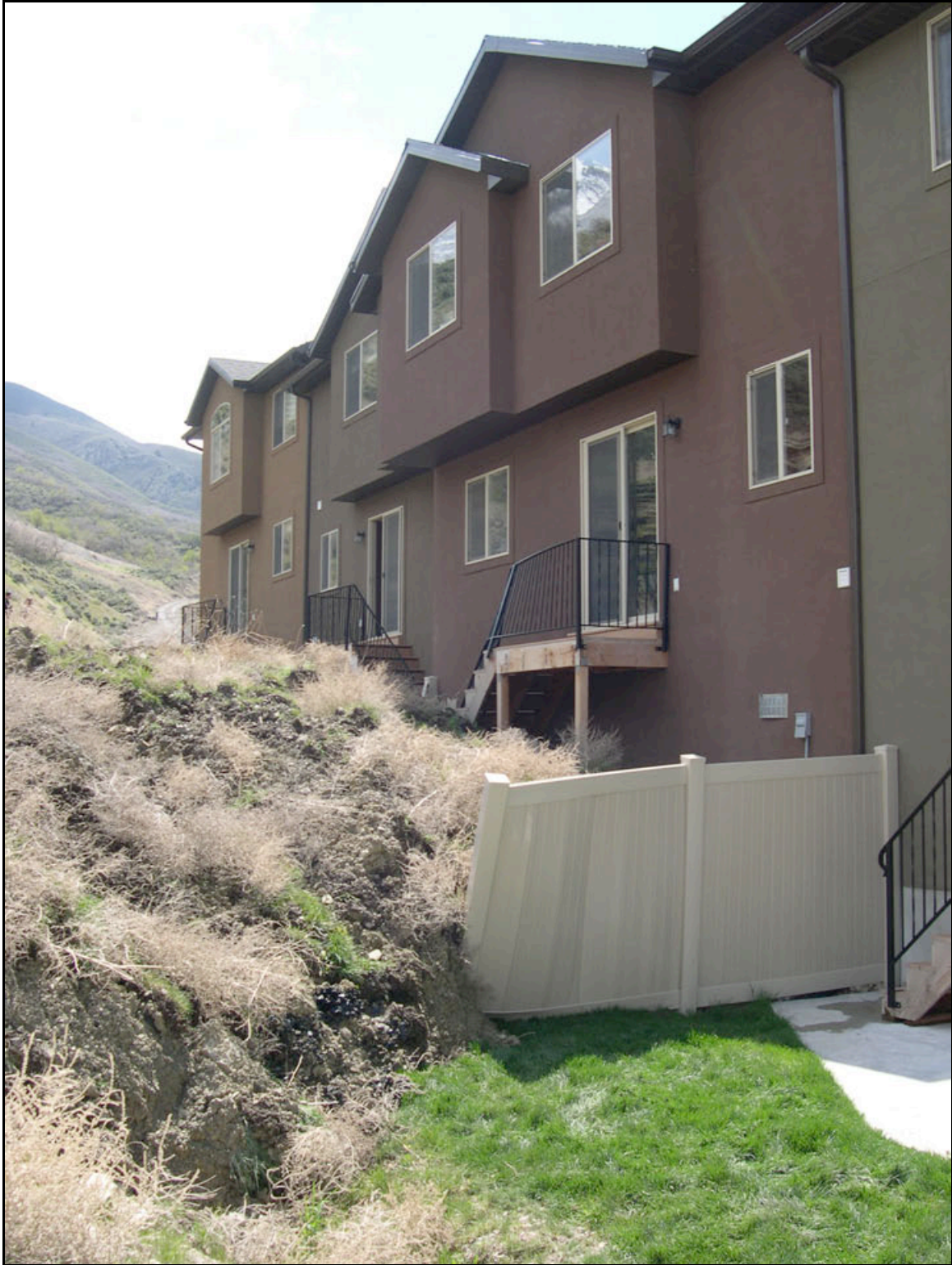
Figure 5. View of the disrupted soil at toe of the landslide and damage to back of townhouse on April 29, 2005.
