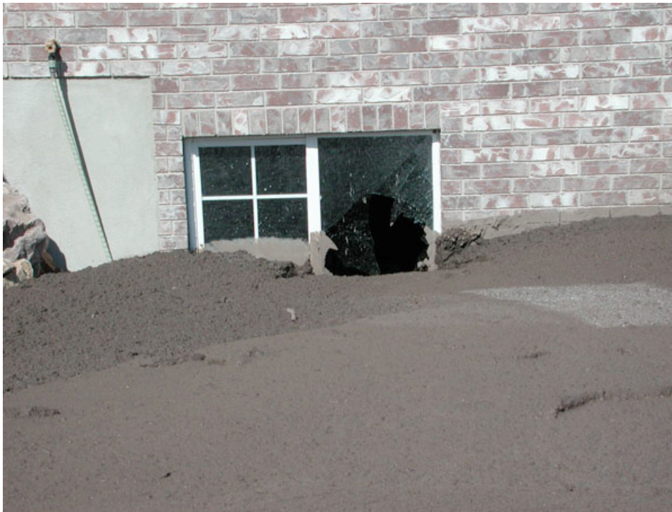
(b) The debris-flow impact broke through this basement window of a house on Apple View Street.
