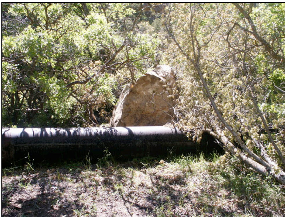
Figure 9. Approximately 13-ton rock-fall boulder, which stopped just before striking the Parowan City penstock.
