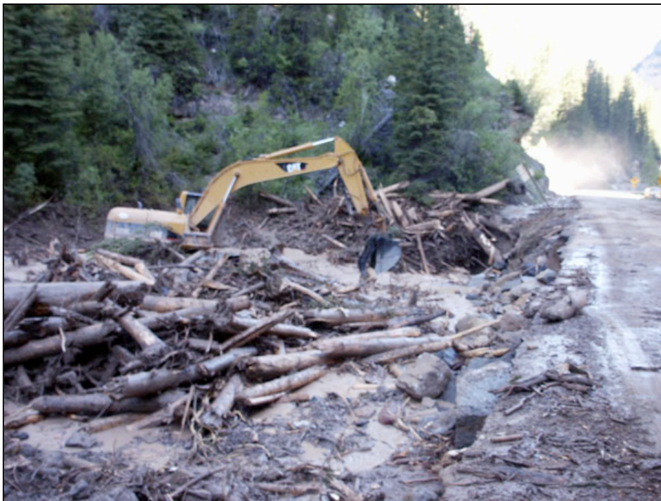
Figure 3. Log jam created by the Black Mountain debris flow at a box culvert beneath SR-14.
