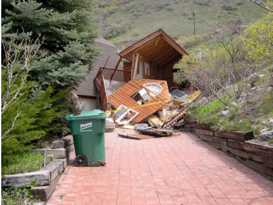
Figure 3. Damage to the guest house. The damaging rock is on the left behind the trash can, against the base of the tree. Parts of the concrete house foundation are behind and to the right of the trash can.
