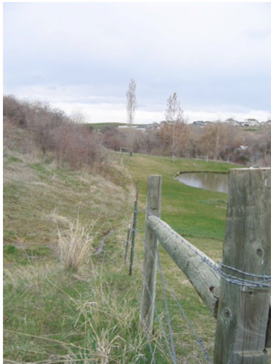
Figure 2. View west of fence displaced by landslide movement in lower slope north and downslope of 1681 East Hillsboro Drive. Photograph taken on April 10, 2006.
