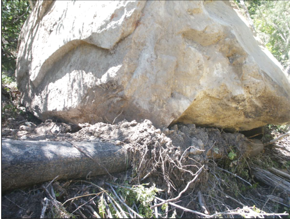
Figure 6. Approximately 80-ton boulder resting on top of the 26-inch diameter Parowan City penstock pipe.
