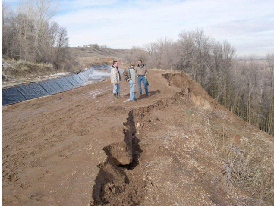
Figure 5. View west of the landslide crown, the Davis-Weber Canal, and the landslide main scarp. Eastward extension of the main scarp in the foreground indicates movement in the slope east of the landslide.
