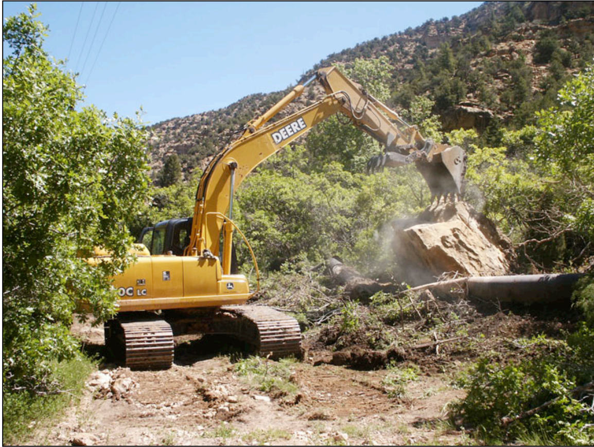
Figure 10. Trackhoe removing the 80-ton boulder from on top of the Parowan City penstock.
