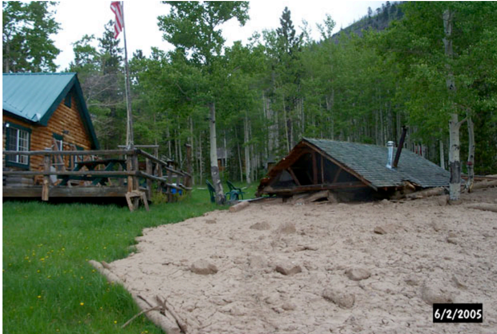
Figure 2. The roof of the Chepta cabin lies on the toe of the U-Bar Ranch debris-flow deposit. The cabin roof is approximately 180 feet downslope of the original cabin position. The U-Bar Ranch lodge (building with green metal roof) is left of the deposit. Photo by Dave Herron, U.S. Forest Service.
