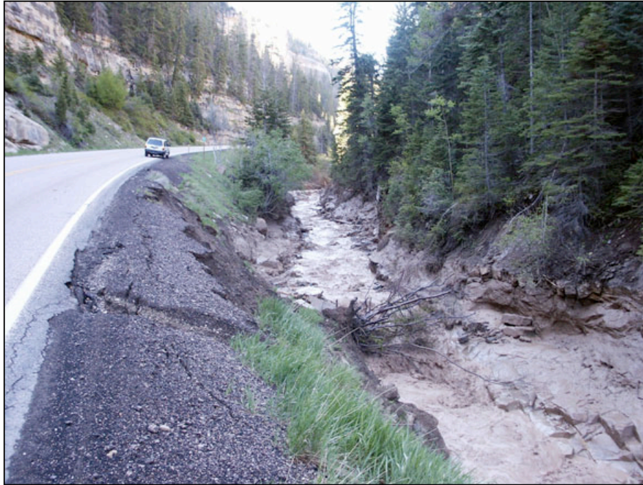
Figure 4. Small slope failure in the roadbed of SR-14 caused by undercutting and erosion of the stream bank by the Black Mountain debris flow.
