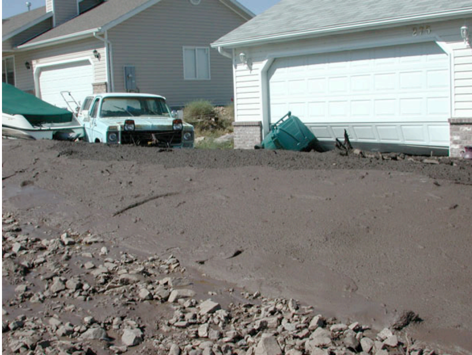
(c) Debris-flow damage to garage doors of house on Peach Street.
