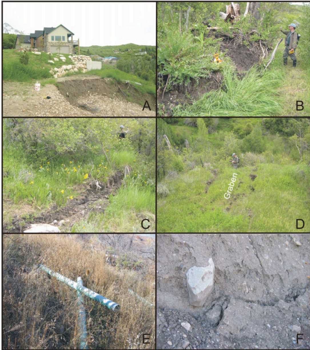
Figure 3. Southern Sewer-Line landslide. (A) View to the northwest of main scarp of the Southern Sewer Line landslide. Landsliding destroyed the eastern part of the sewer corridor embankment, but had not exposed the sewer pipe as of January 13, 2006. House at 6110 N. Creekside Drive visible in background. (B) View to the northwest of toe of the landslide. Lower toe thrust/fold is approximately 5 feet high. West edge of Gordon Creek (not visible just to the right of the edge of the photograph) was only 3.4 feet from toe on October 12, 2005. (C) View downslope of right-flank shear cutting across natural slope. (D) View downslope of east-trending graben in lower part of slide. (E) Broken drainpipe in lower part of slide. Upslope pipe displaced about 3.9 feet downslope. (F) Recent offset of main scarp on November 1, 2005, due to continued movement of slide in latter part of 2005.
