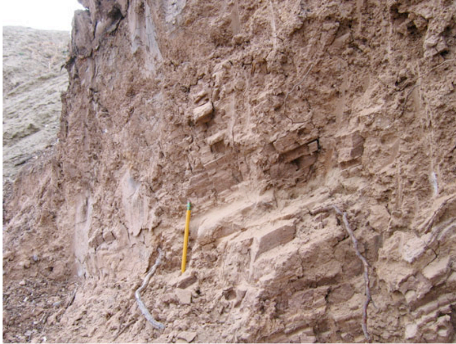
Figure 1. View of cut slope at 1681 East Hillsboro Drive showing tilted Lake Bonneville sediments. The bedding strikes N. 65° W. and dips 38° NE. Photograph taken on November 11, 2005.
