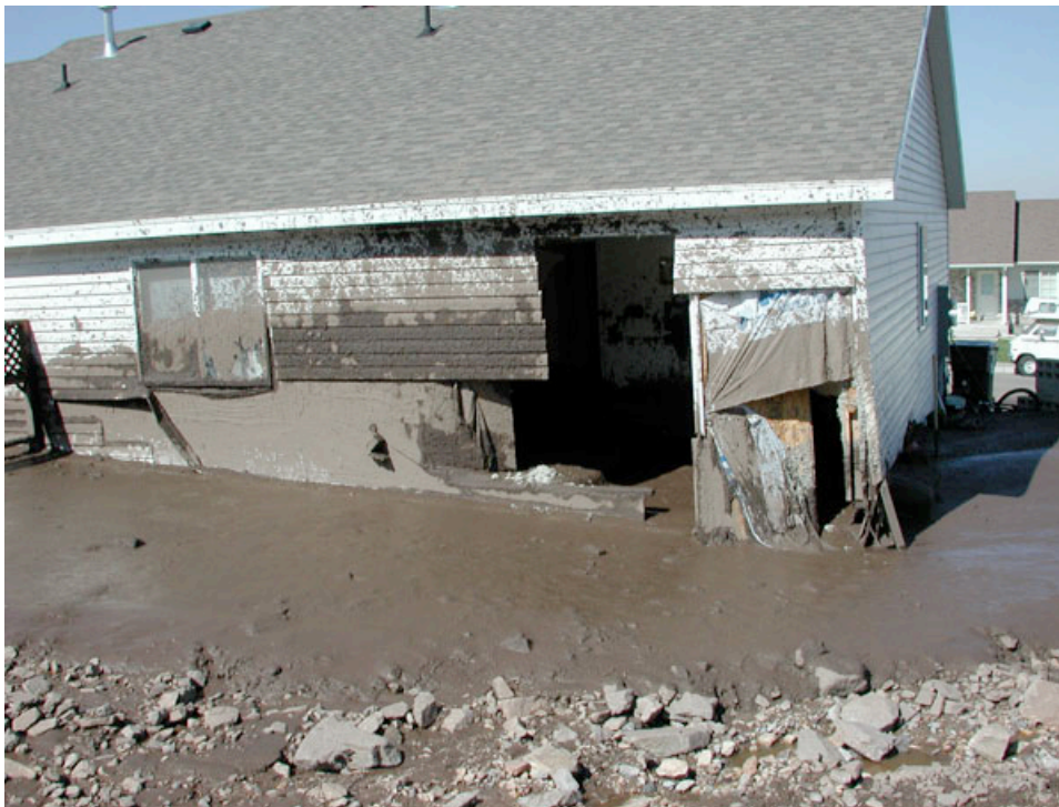
(d) Debris-flow damage to the back wall of house on Peach Street.
