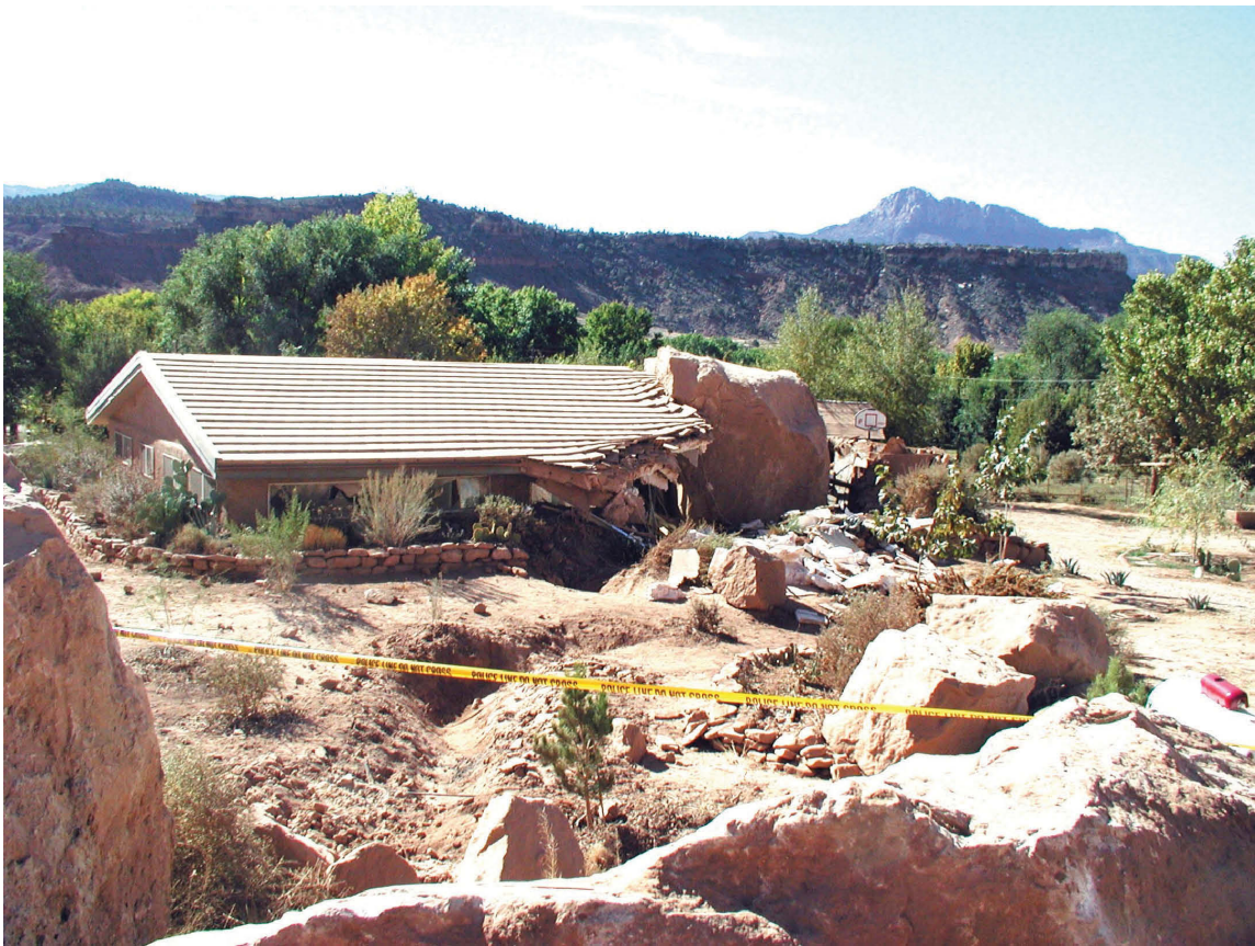
Figure 14. Rockville home at 200 North Center Street struck by an estimated 300-ton rock-fall boulder on October 18, 2001. Photo courtesy of Bill Lund.
