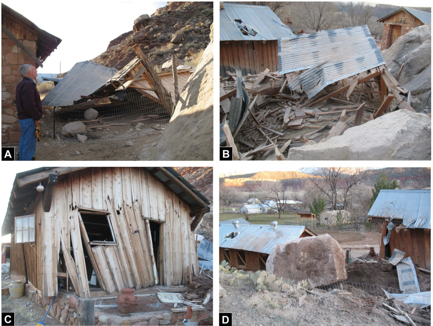
Figure 5. Damaged outbuildings at 274 West Main Street; photos taken on February 10, 2010. A., B. Destroyed sheds adjacent to impact area. C. Damaged workshop knocked off its foundation. D. Largest (9 x 6 x 5 feet) post-impact boulder that damaged a workshop (right) and shed (left).
