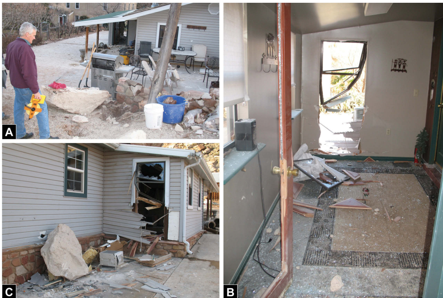
Figure 6. Rock-fall damage to the house at 274 West Main Street; photos taken on February 10, 2010. A. View downslope along path of the rock that damaged the house. Narrowly missing a barbecue grill, the rock rolled through the entryway and mudroom on the left (east) side of the house. B. Looking through the mudroom where the boulder broke through a glass door, which is still on its hinges, and exited through an exterior wall and window. C. After exiting the mudroom, the rock collided with a parked car and came to a rest. The rock, estimated to be 3.5 x 3 x 1.7 feet, was later moved up against the house when the damaged car was moved.
