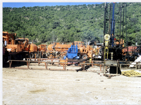
Completing the Chasel 3-6A2 well.
