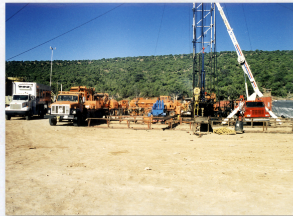
Completing the Chasel 3-6A2 well. Preparing to acid treat the well.
