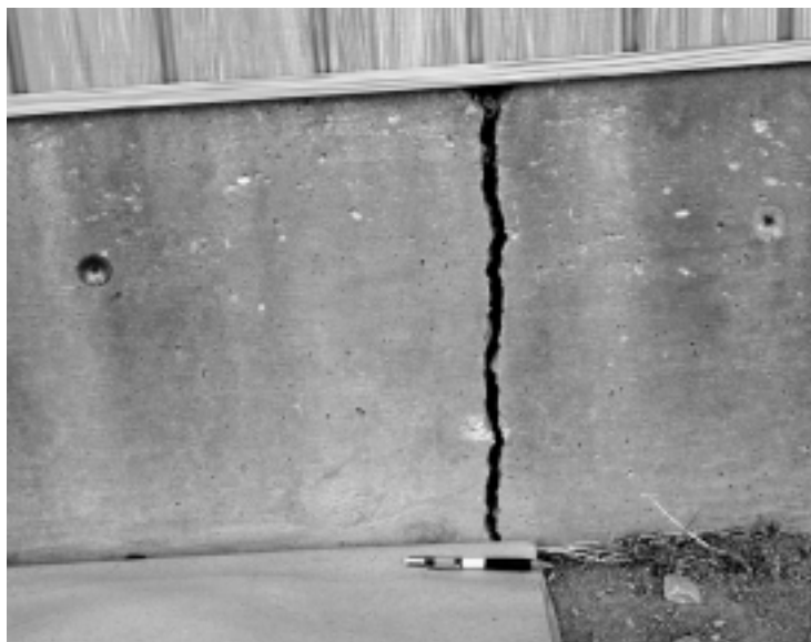
Figure 5. Typical crack in concrete foundation wall due to soil collapse on the Sand Canyon alluvial fan southeast of the Sand H debris basin.
