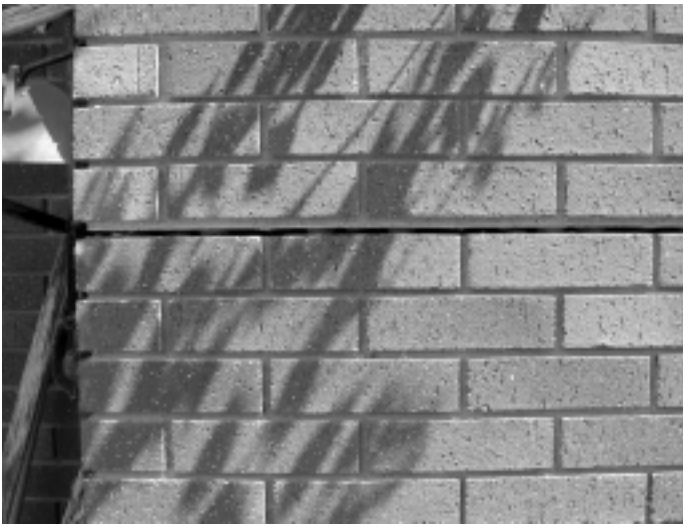
Figure 6. Crack developed along mortar in brick wall due to soil collapse on the Sand Canyon alluvial fan southeast of the Sand H debris basin.
