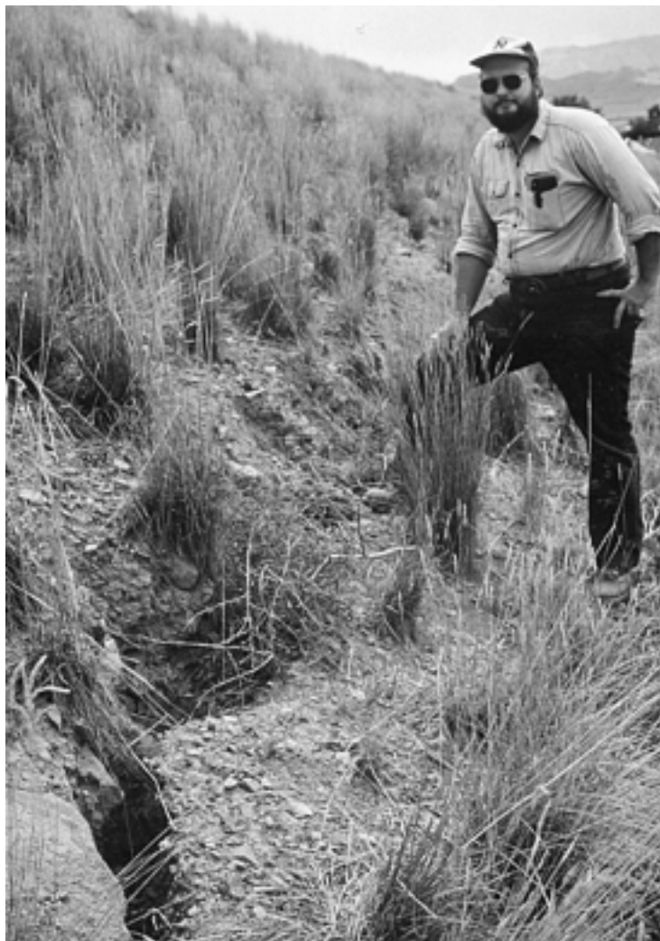
Figure 4. Crack developed in the Sand H debris basin embankment due to soil collapse (from U.S. Soil Conservation Service, 1984).
