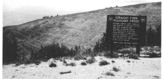
Figure 4. Forest Service-terraced land to retard erosion until protective vegetation cover becomes established.
