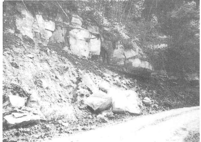
Figure 5. Rock fall hazard due to road cut in Straight Fork of Pleasant Creek.
