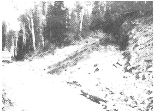
Figure 6. Slope failure due to road cut near North Fork Creek.
