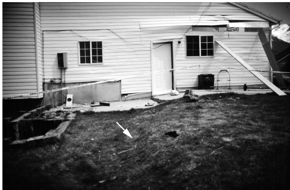
Figure 5. Damage to house on lot 105 at the Sunset Drive landslide in Layton. View of west side of house showing severe damage. Main scarp of the landslide is visible in foreground (arrow).
