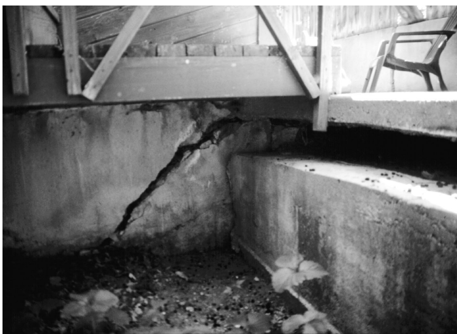
Figure 20. Foundation damage to a house at the Springhill landslide. View of southwest corner of house.
