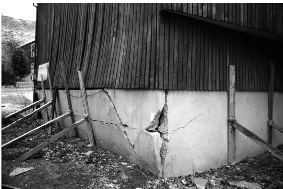
Figure 3. Condemned house at the Springhill landslide in North Sale Lake prior to demolition. View of northwest corner of house showing severe foundation damage.
