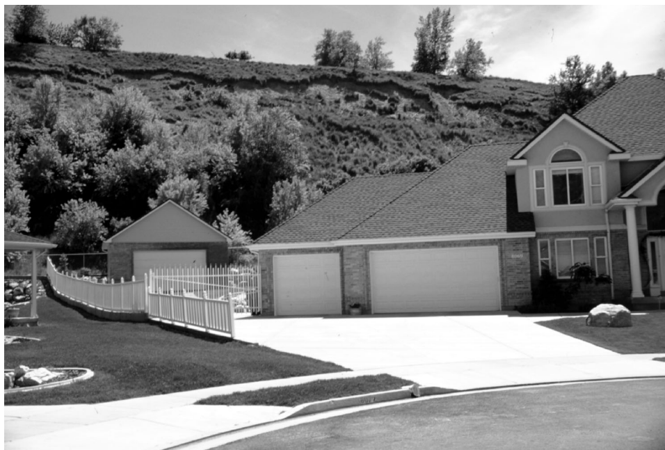
Figure 15. Shallow earth-slide complex at the Cedar Bench Subdivision landslide. View is toward the southwest.
