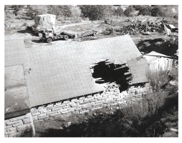
**Figure 3.1.** Damage to the roof of the Zion National Park maintenance facility in Oak Canyon caused by a rock-fall boulder in 1946 (photo courtesy of the National Park Service).
