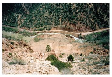
Figure 4.5. Temporary road graded around the Sentinel landslide, April 1995 (photo credit G.F. Wieczorek, U.S. Geological Survey).
