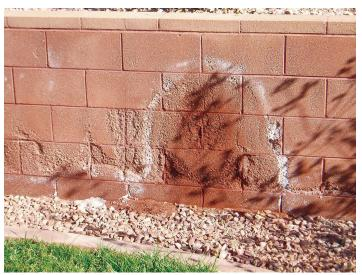
**Figure 6.6.** Corrosion of masonry block walls in southwestern Utah due to the reaction of the non-Type V cement used in the masonry blocks with high-sulfate soils (photo credit David Black, Rosenberg Associates).
