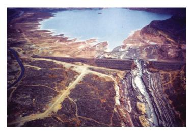
**Figure 6.5.** Quail Creek dike failure, January 1, 1989, in southwestern Utah was due in part to gypsum dissolution in the underlying Shnabkaib Member of the Moenkopi Formation (photo credit Ben Everitt).
