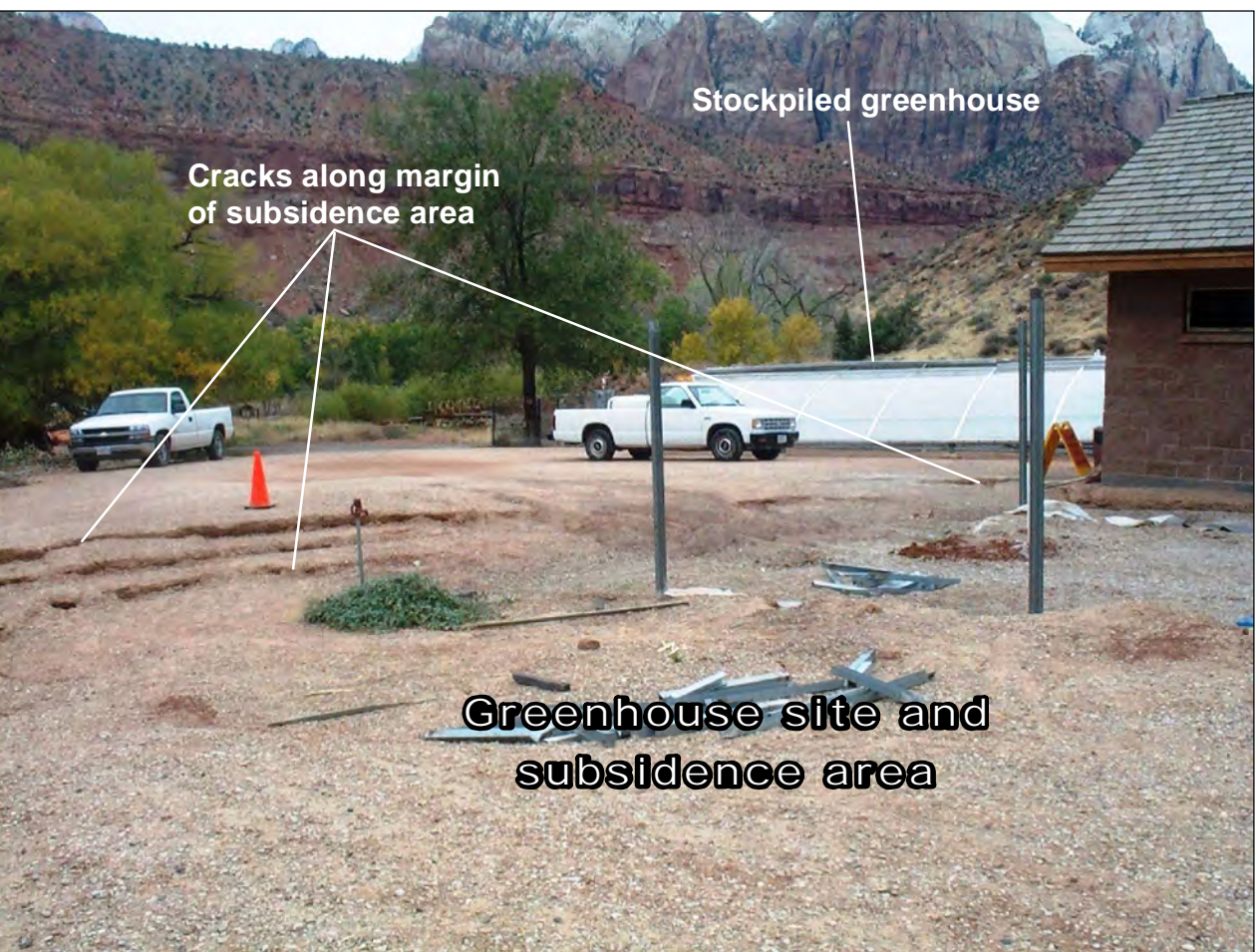
Figure 2. Site of the Zion National Park greenhouse (stockpiled behind truck near photo center) damaged by collapsible soils. Circa 2001 photo; courtesy of the National Park Service.
