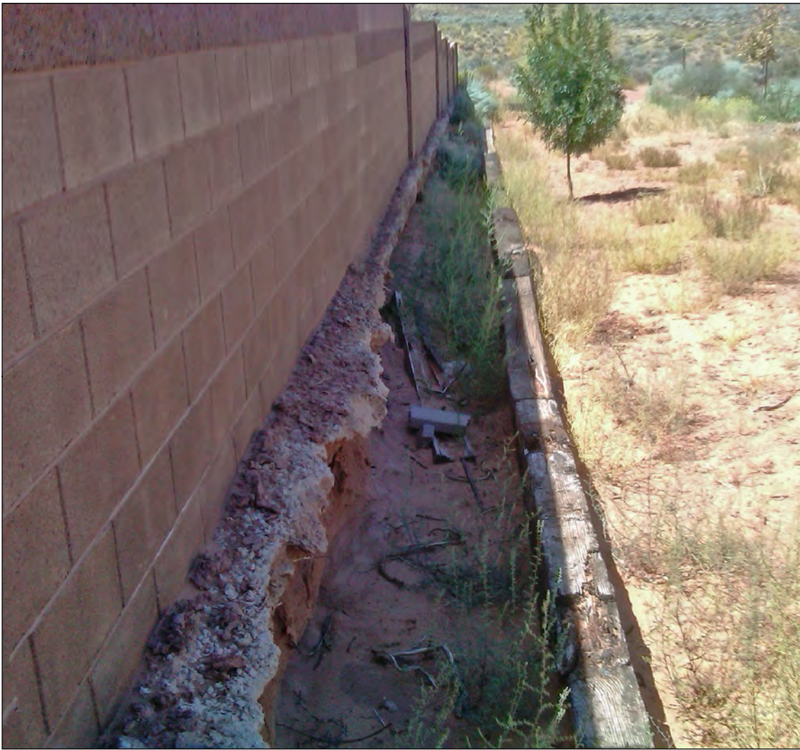
Figure 4. Exposed block wall foundation in Virgin due to wind erosion of sandy soil (photo credit David Black).
