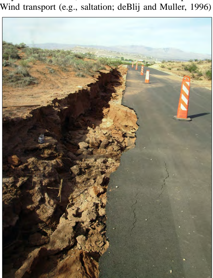
Figure 3. Gully formed in fine-grained material during a cloudburst thunderstorm in southwestern Utah. Photo date: February 2006.
