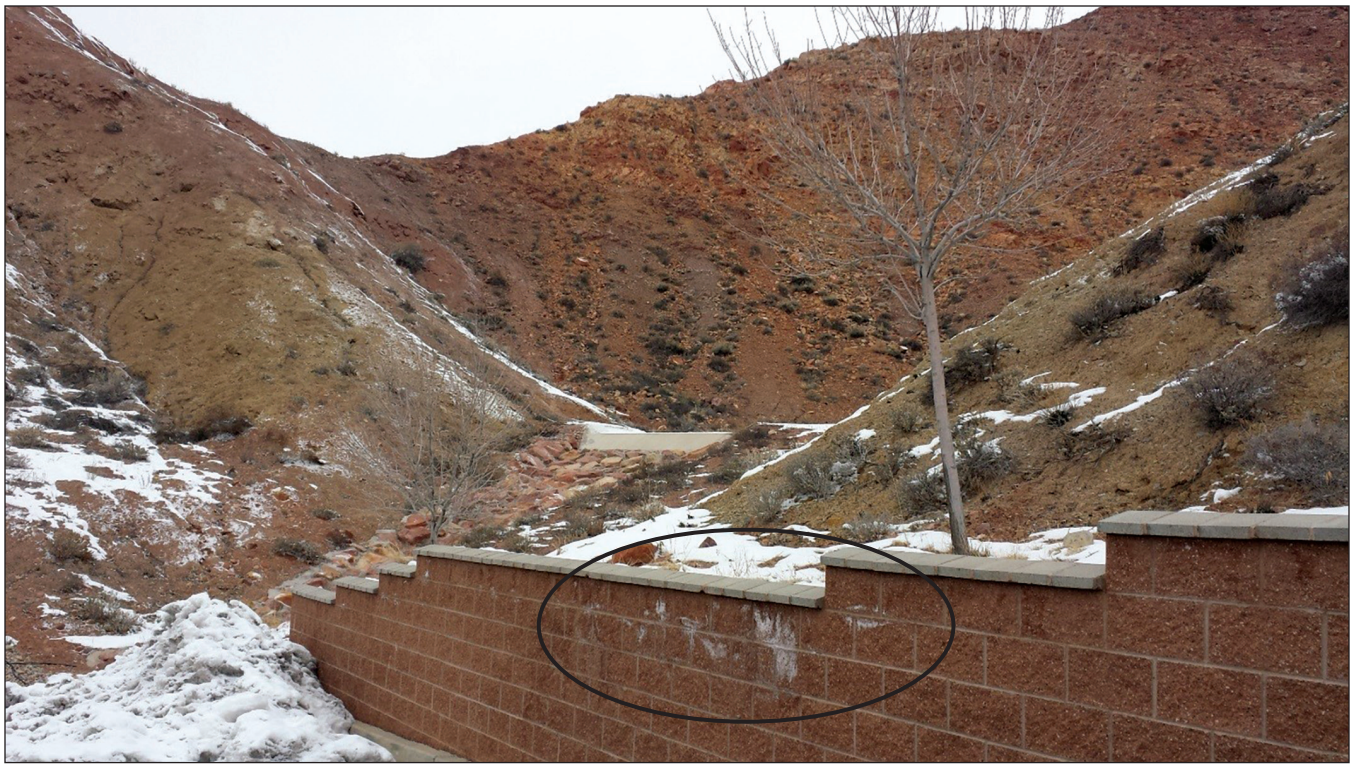
Figure 14. Evaporite precipitation and corrosion on concrete masonry unit wall (photo: northeast valley margin, February 23, 2017).
