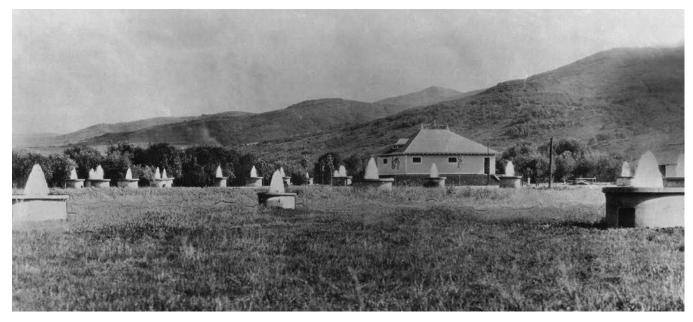
Figure 5. Flowing wells at Artesian Park near the head of Ogden Canyon. The wells provided water to Ogden City beginning in 1914 and were either plugged or extended to the current location of Ogden City well field before the area was inundated by Pineview Reservoir in 1937. All wells were eventually plugged and new supply wells were drilled. Photo credit: Utah State Historical Society, used with permission.
