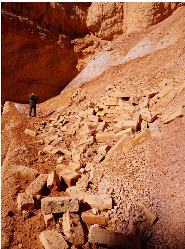
Figure 13. Damage to the Navajo Loop Trail due to shallow landsliding in the Claron Formation. Such shallow landslides are commonly associated with modifications made to the natural slope during trail construction. Photo taken April 3, 2020.
