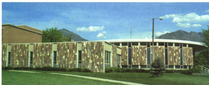
Figure 7. Stone veneer at Olympus High School, 4055 South 2300 East, Salt Lake City, Utah. Veneer stone is mixed sandstone and quartzite laid in a "planking" pattern.
