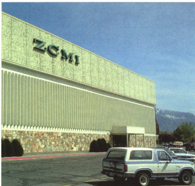
Figure 9. Stone veneer at the ZCMI building (Cottonwood Mall), 4835 South Highland Drive, Holladay, Utah.
