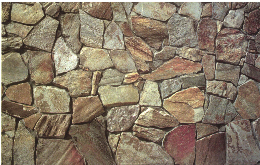
Figure 10. Close-up of veneer stone at ZCMI building.
