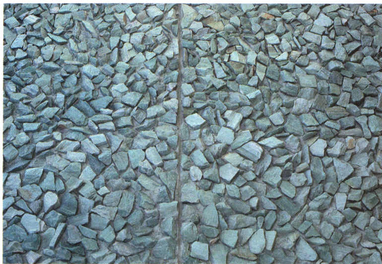
Figure 13. Close-up of crushed Elba Quartzite used in precast panels on a building, 530 East 400 South, Salt Lake City, Utah. Individual "chunks" average 3 inches (8 cm) in diameter.
