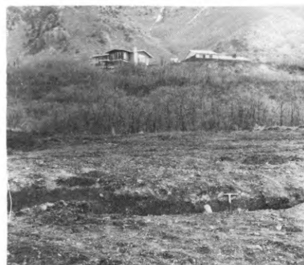
March 17. Uppermost scarp was planed off and crevasses filled in; scarp grew 16 inches the next 24 hours and averaged 18 inches per day the next week.
