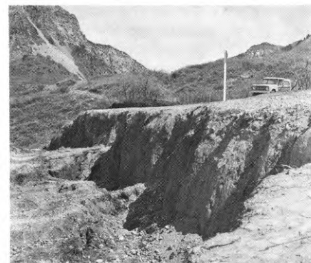
March 27. Nine days after the scarp area had been bulldozed to a flat surface, the scarp height measured 14½ feet.
