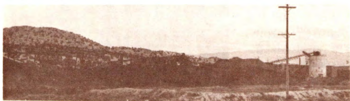
(6) Utah International, Inc. 's stockpiled iron ore and conveyor belt at the Iron Springs district facility. The Iron Springs district is the largest iron-producing district in the western states. In 1971 approximately 291,000 tons of ore were produced. Ore bodies lie 12 to 20 miles west of Cedar City.
