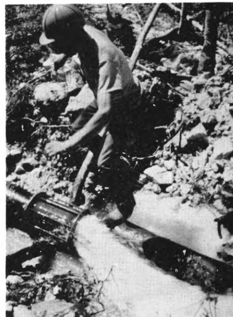
Above: Scarp formed by earth movement beginning May 26, 1974. View is south, toward head of the slide area. Right: Offset in waterline caused by the May, 1974, earth movement.
