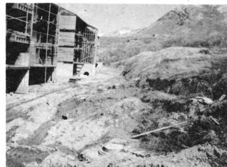
New apartments are under construction on an old landslide at mouth of Ogden Canyon. Such developments have prompted solicitation of an opinion from the Utah Attorney General's office on the state's responsibility. Note active sliding in foreground on recently created cut-slope.
