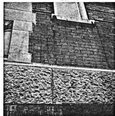
Left: Storage bin spilling barley. Note severe buckling and shifting on concrete foundation, an indication of intense ground shaking. Evidence for both vertical (1 inch) and horizontal (2½ inches) ground motion was observed. (UGMS photo) Top Right: Epicenter located in southern Idaho. Bottom Right: Cracks in front of Sumner School, Salt Lake City. Some bricks were displaced higher on the wall. (UGMS photo)
