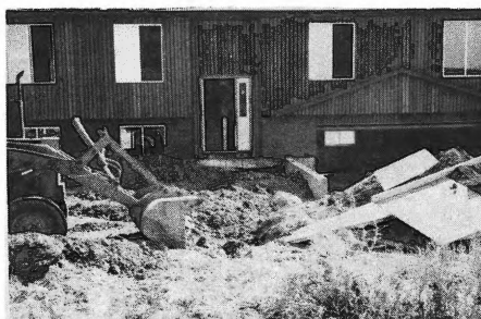
Collapsed and back-filled trench at homesite north of Riverton, Utah.
