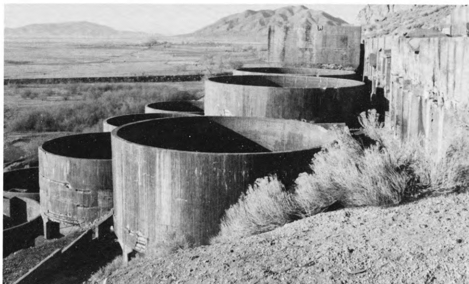
FIGURE 5. The complex mineralogy of Tintic ores led to many metallurgical experiments. This chloridization roasting/leaching plant east of Goshen, just south of the highway to Tintic, is a colorful reminder of the old Tintic Standard, once the richest silver mine in the world. L. P. James photo.
