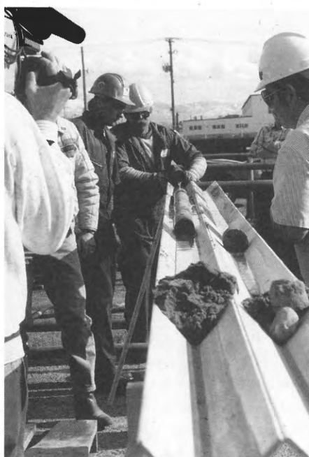
The inner barrel containing the core is laid on the pipe racks. The core is forced out with water onto a core tray where it can be measured and described.
