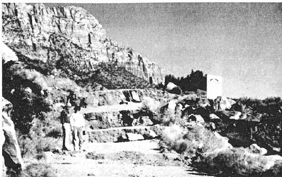
Landslide scarps deform gravel road in the Balanced Rock Hills Subdivision in Springdale. The landslide was triggered by the September 2, 1992 St. George Earthquake. (photo by UGS staff)
