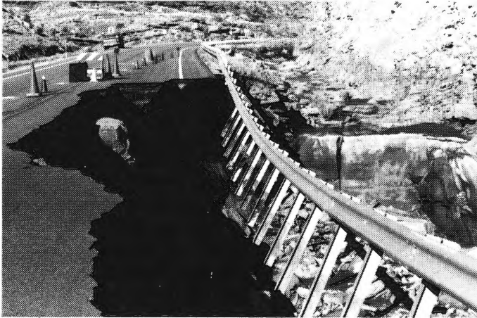
U. S. Highway 191 damage with the water gap to the right. Note the shallow channel which normally carries runoff without overflow (photo by Paul Guardy).
