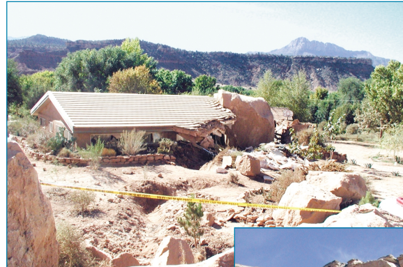
▲ Home in Rockville, Utah struck by a boulder that dislodged from an adjacent cliff. Note the gouge where boulder bounced across the yard.
