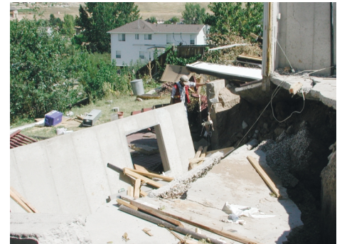
Basement and foundation straddling the main scarp. The wood frame portion of the house was moved off the foundation on August 25, 2001.
