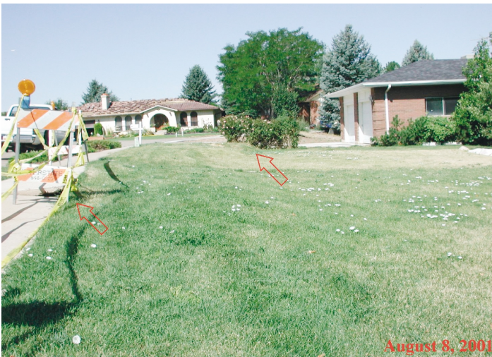
In the left photograph the arrows point to the tilted sidewalk (left) and roll in lawn (right) showing small main-scarp displacements on August 8, 2001. In the right photograph the arrows point to the same locations showing main-scarp displacements of 4 to 5.5 feet on August 27, 2001.
