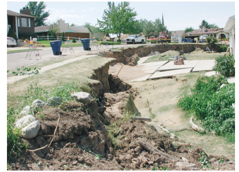
Lawns, driveways, and sidewalks displaced by the broad, curving main scarp up to 5 feet high.
