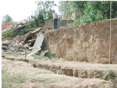
Main scarp height of 9 feet with the remains of demolished house at left. Note the displacement increase from photo above.
