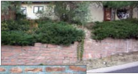
Both of these walls are built with Nugget Sandstone; the left wall uses random shapes and sizes floated in mortar, while the wall on the right uses tightly fit, hand-hewn blocks.
