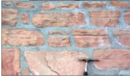
Both of these walls are built with Nugget Sandstone; the left wall uses random shapes and sizes floated in mortar, while the wall on the right uses tightly fit, hand-hewn blocks.
