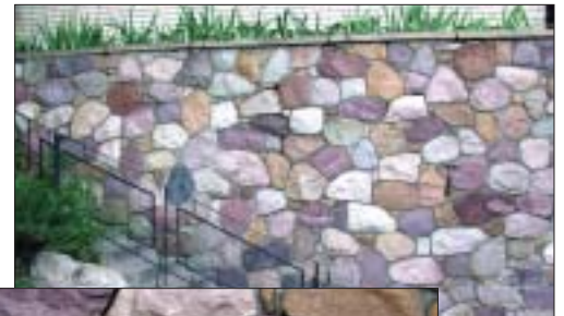
The stone on both of these walls is not structural, but a thin veneer. The right wall is veneered with split-face quartzite fieldstone. Part of a new conference center in downtown Salt Lake City, the left wall is clad in cut granitic blocks from Little Cottonwood Canyon (Salt Lake County).
