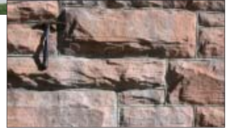
Both of these walls are built with Nugget Sandstone; the left wall uses random shapes and sizes floated in mortar, while the wall on the right uses tightly fit, hand-hewn blocks.
