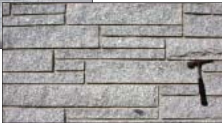
The stone on both of these walls is not structural, but a thin veneer. The right wall is veneered with split-face quartzite fieldstone. Part of a new conference center in downtown Salt Lake City, the left wall is clad in cut granitic blocks from Little Cottonwood Canyon (Salt Lake County).
