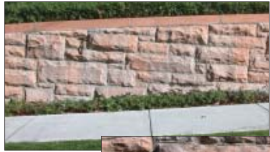
Both of these walls are built with Nugget Sandstone; the left wall uses random shapes and sizes floated in mortar, while the wall on the right uses tightly fit, hand-hewn blocks.
