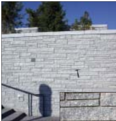
The stone on both of these walls is not structural, but a thin veneer. The right wall is veneered with split-face quartzite fieldstone. Part of a new conference center in downtown Salt Lake City, the left wall is clad in cut granitic blocks from Little Cottonwood Canyon (Salt Lake County).
