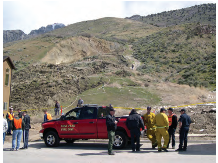
Damaged townhouse and disrupted toe and main scarp of the landslide in Cedar Hills.
