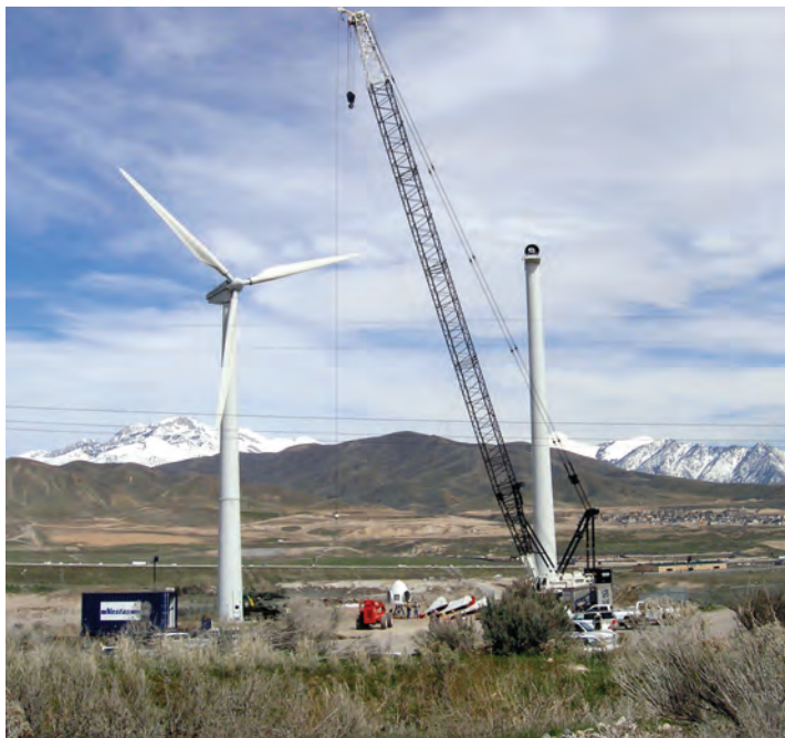
A new 665 kilowatt turbine is installed next to the original 225 kilowatt turbine at Camp Williams. Photo by Mike Vanden Berg.
