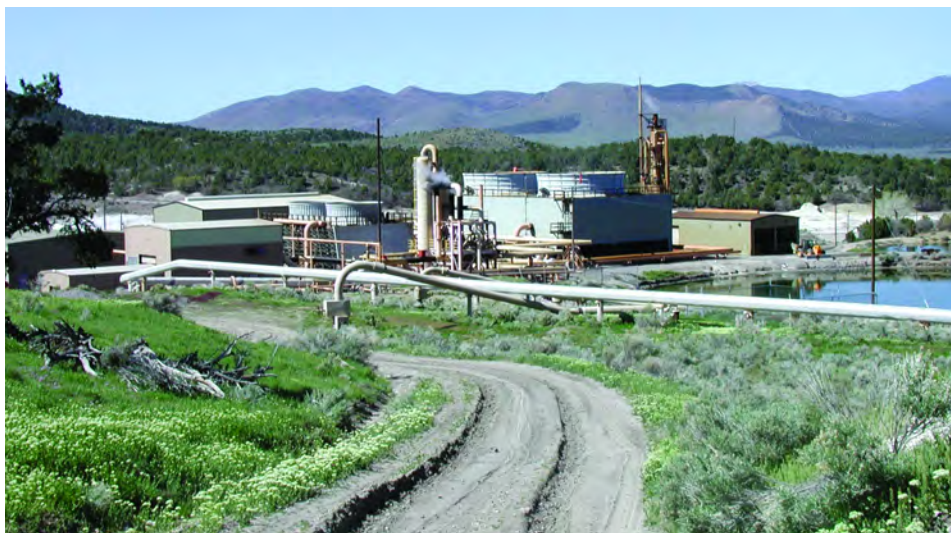
Geothermal power plant at the Cove Fort-Sulphurdale geothermal area near the I-70 – I-15 junction, Millard and Beaver Counties, Utah. Amp Resources is proceeding with exploratory and development drilling in anticipation of reconstructing the plant into a 37 MW Kalina-cycle facility.
